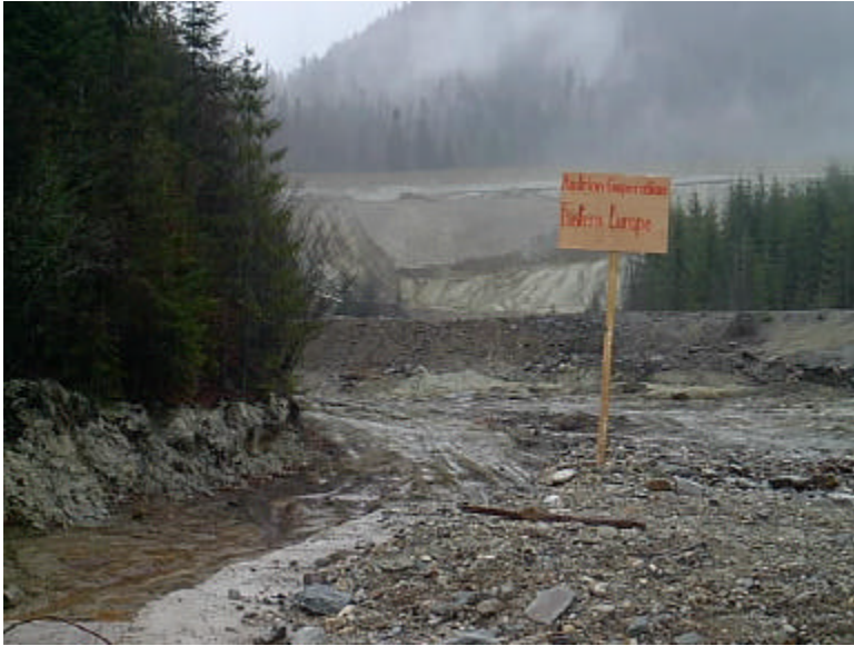
Upstream view from the exfiltration pond: The tailings deposited here after the accident in March 2000 were moved out (upstream) in order to increase the pond's capacity for collecting seepage water of the tailings pond.
