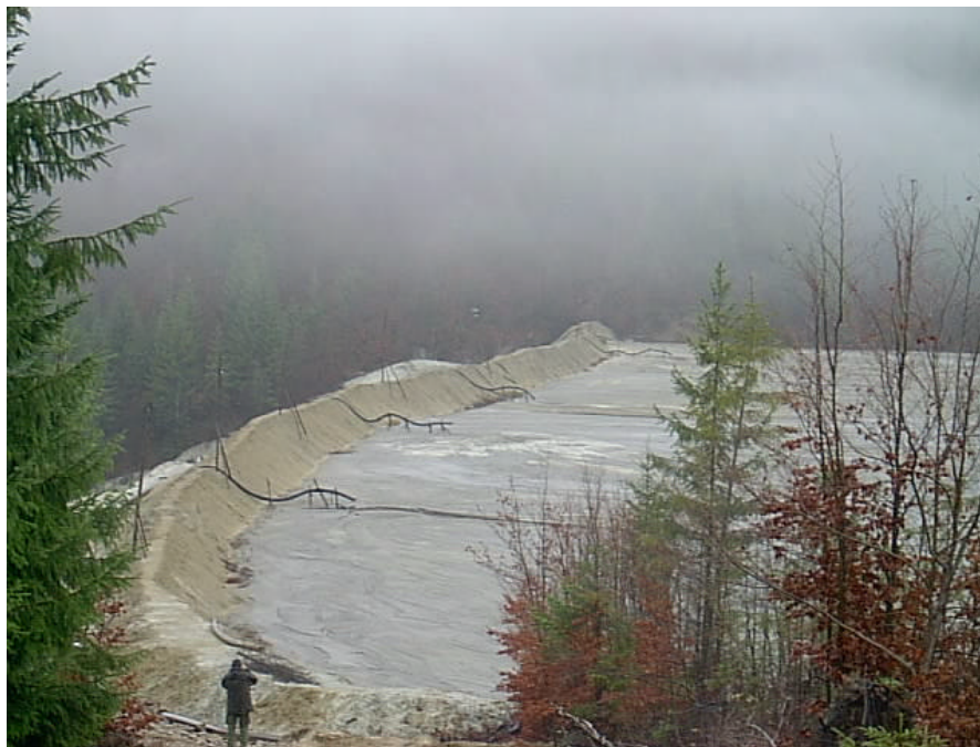
View to the main tailings pond (with the raised crest for increased freeboard at left and the expanded beach at right)
