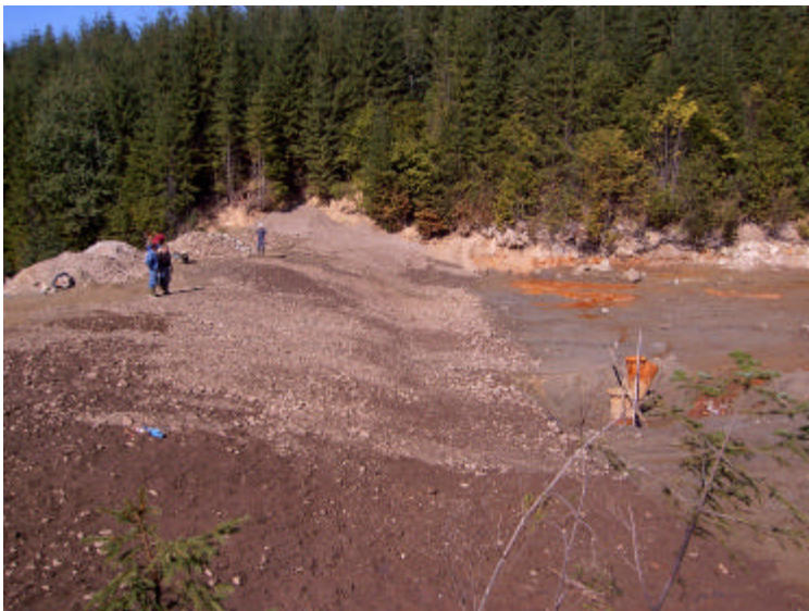
Exfiltration pond: The embankment was re-shaped and made water-tight with a geo-membrane (photo on top). A new emergency spillway was built on the central section of the dam (photo below).
