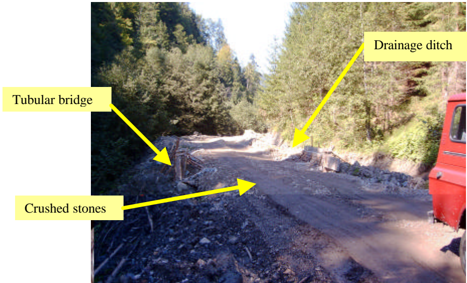
The mountain road from Baia Borsa to the Novat valley is in a very bad state (photo by Zinke on top from July 2004) and could be partly repaired during the project (especially in the lower section near the tailings pond: photo: Horvath).
