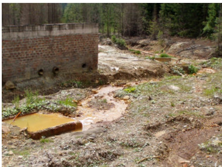
The pumping station of the exfiltration pond was mostly destroyed by the March 2000 accident and only re-built in 2004. At the left bottom (see both the photo on top from July 2004 (by Zinke) and the photo below from early November 2004), the outlet of the pond (penstock) still discharges contaminated seepage water around the house into Novat creek.
