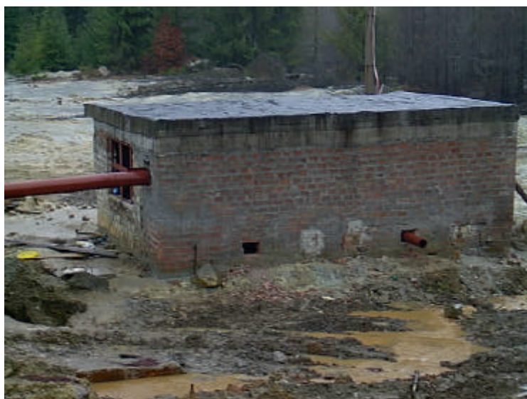
The pumping station of the exfiltration pond was mostly destroyed by the March 2000 accident and only re-built in 2004. At the left bottom (see both the photo on top from July 2004 (by Zinke) and the photo below from early November 2004), the outlet of the pond (penstock) still discharges contaminated seepage water around the house into Novat creek.
