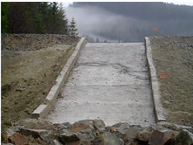
Exfiltration pond: The embankment was re-shaped and made water-tight with a geo-membrane (photo on top). A new emergency spillway was built on the central section of the dam (photo below).
